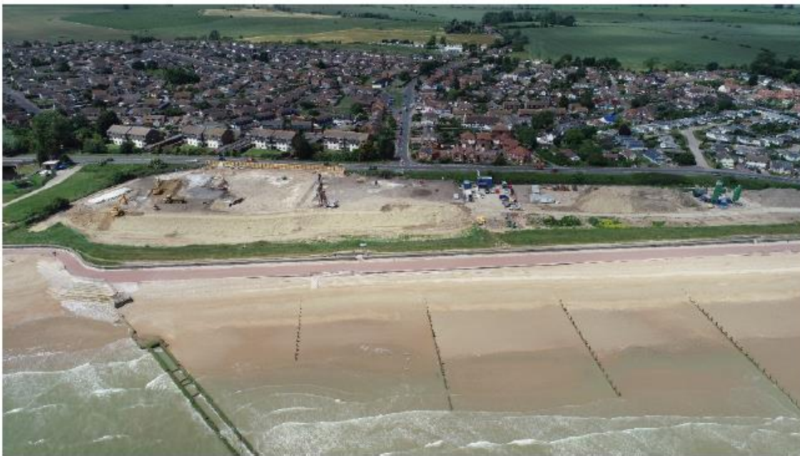
Figure 1 Soil improved ground at Saint Mary's Bay, Kent. Photo courtesy of Deep Soil Mixing
