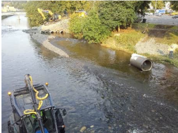
Figure 3: Pipe bridge under construction
