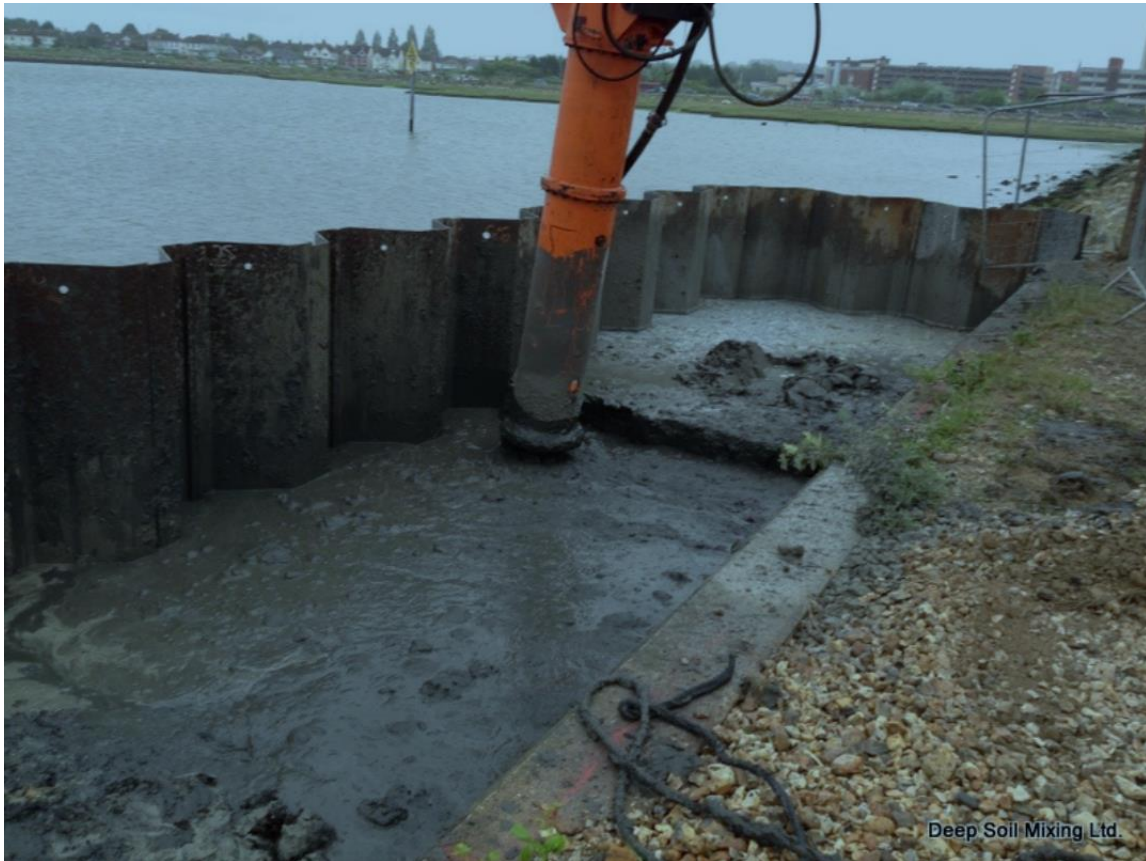
Figure 2 Soil improved ground at Poole. Photo courtesy of Deep Soil Mixing
