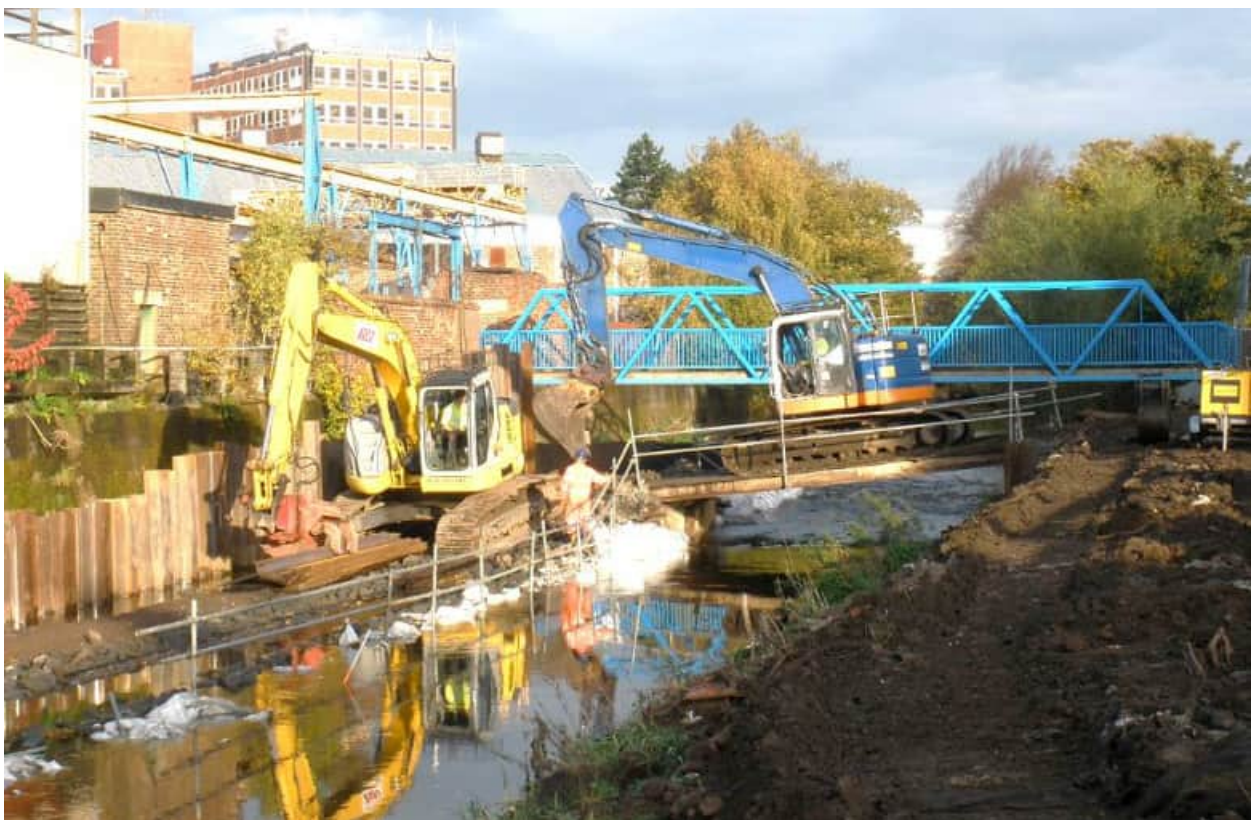
Figure 4: Example of a Bailey bridge in use
