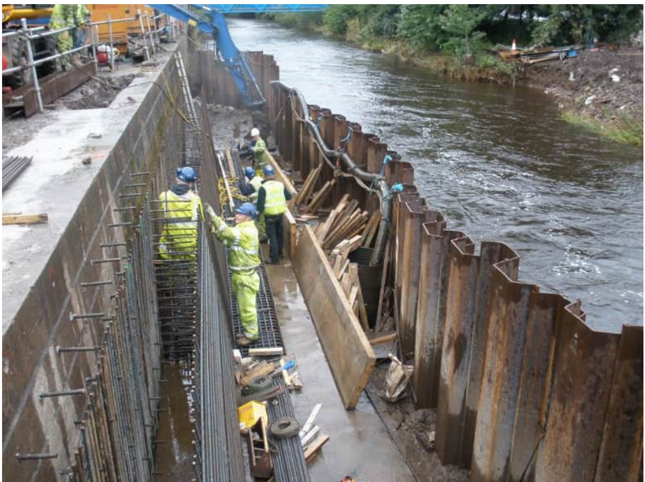
Figure 1: Example of a cofferdam, White Cart Water FPS, Glasgow, 2009
