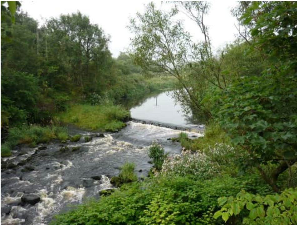
Photograph 13.2 - Weir Carron Iron Works (Asset 18)
