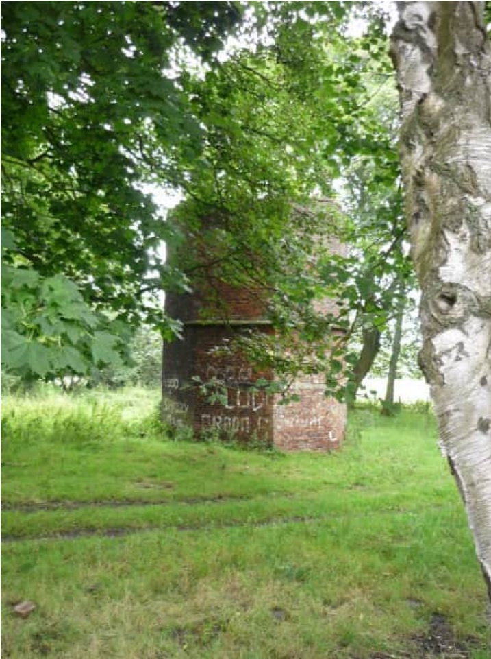
Photograph 13.1 - Dovecot, Carron House (Asset 11)
