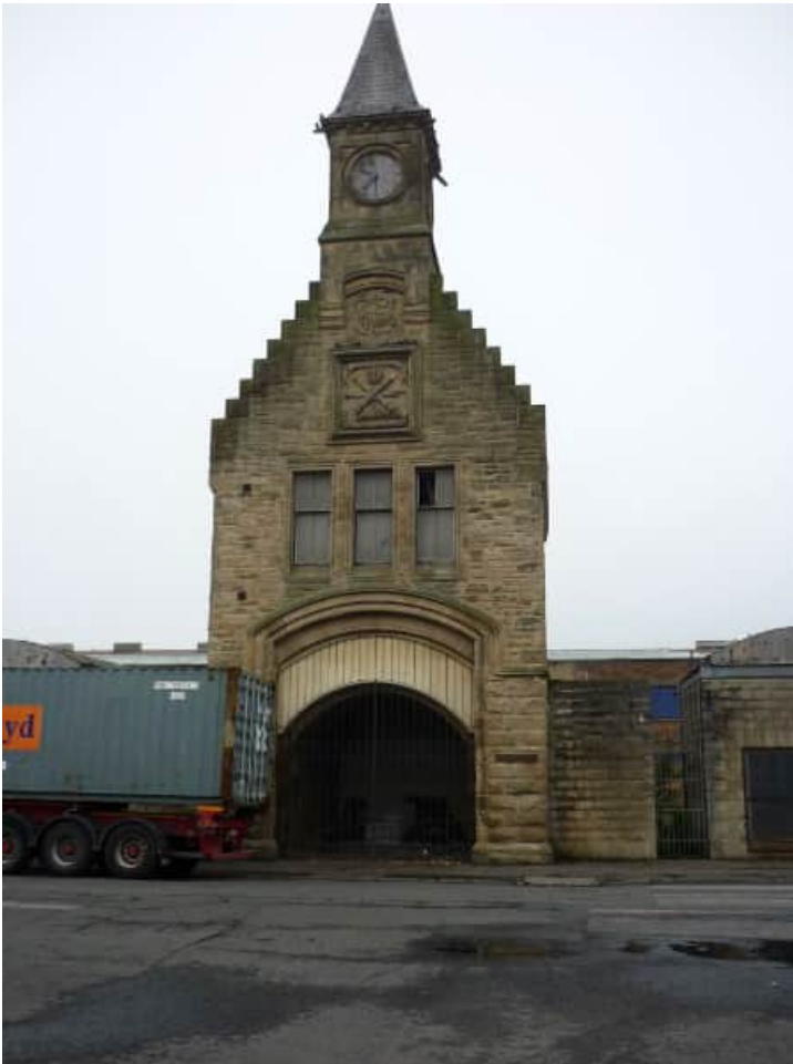
Photograph 13.5 - Carron Company, Clock Tower Remnant of Former Office Block (Asset 16)
