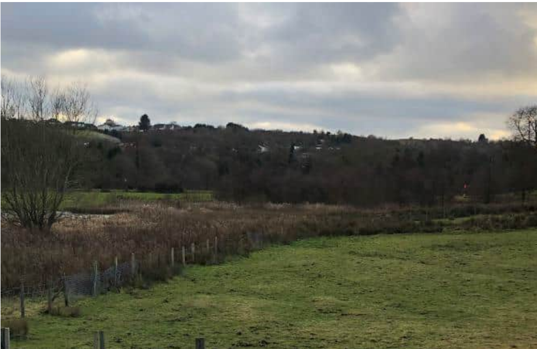
Figure 16: Masts with hi-vis flags showing dam structure
