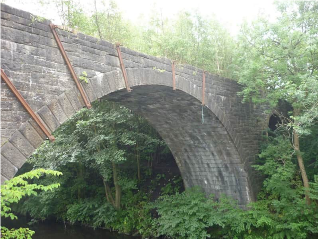
Photograph 13.3 - Former Railway Bridge Across River Carron Iron Works (Asset 19)
