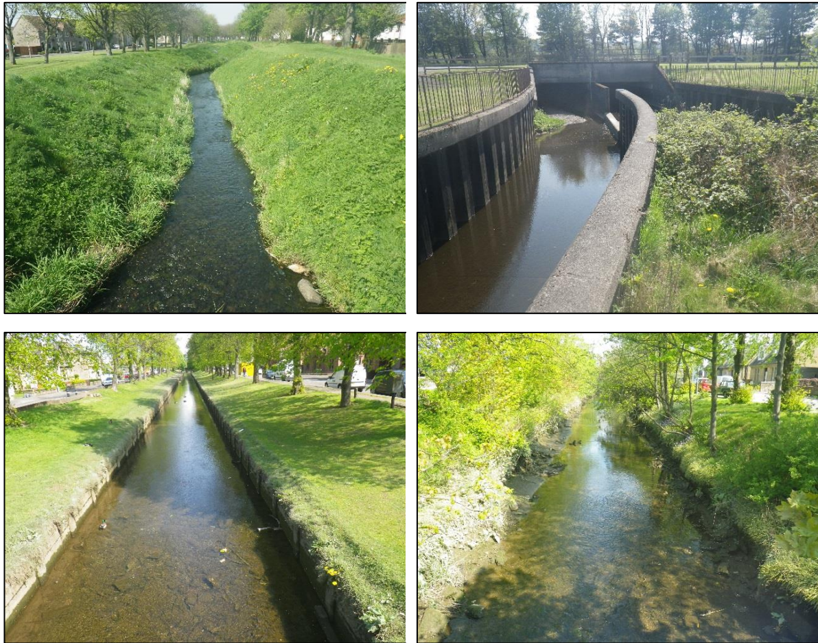
Plates 4.5 – 4.9: Grange Burn: Grassy uniform embankments on floodplain (top left), culverts at upstream section where flood alleviation channel adjoins Grange Burn upstream (top right), Upstream the channel is narrower with wooden toe protection (bottom left). Bank protection is failing in places (bottom right).
