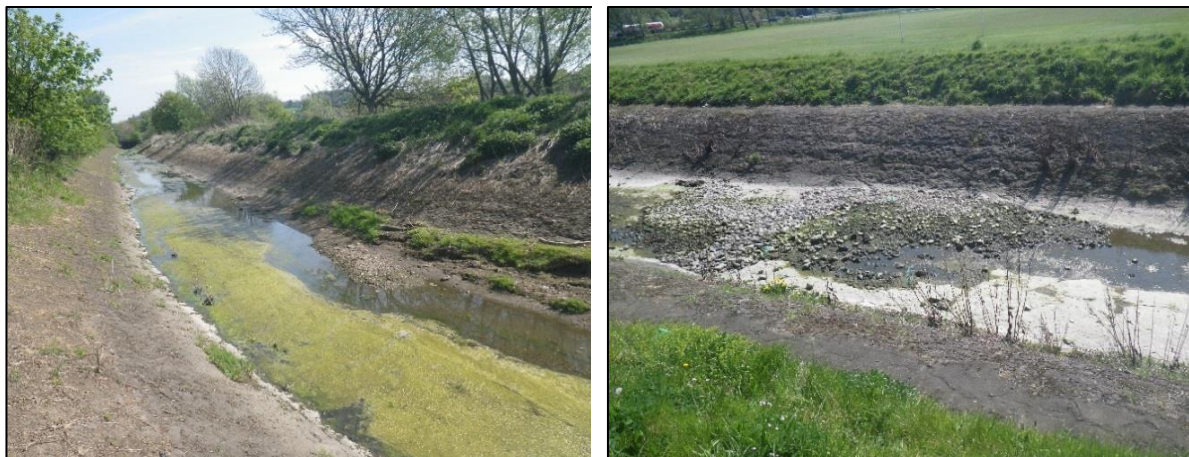
Plates 4.10–4.11: High, uniform trapezoidal shaped embankments with low flow and ponding water under normal flow conditions (left) and localised areas of gravel deposition (right)
