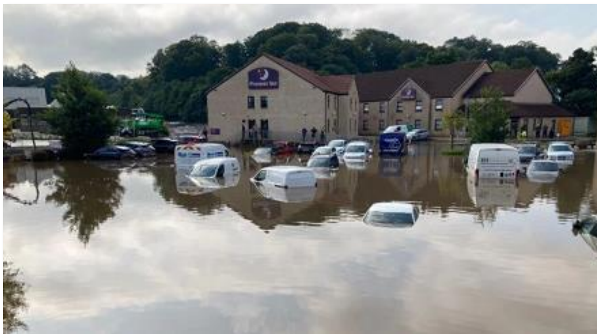
Photograph 1-2: Flooding at Beancross (August 2020)
