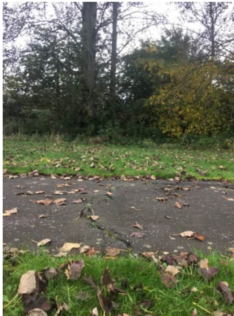
S011019 GFPS Image No 06 Surface damage from Poplar roots on Wholeflats Rd
