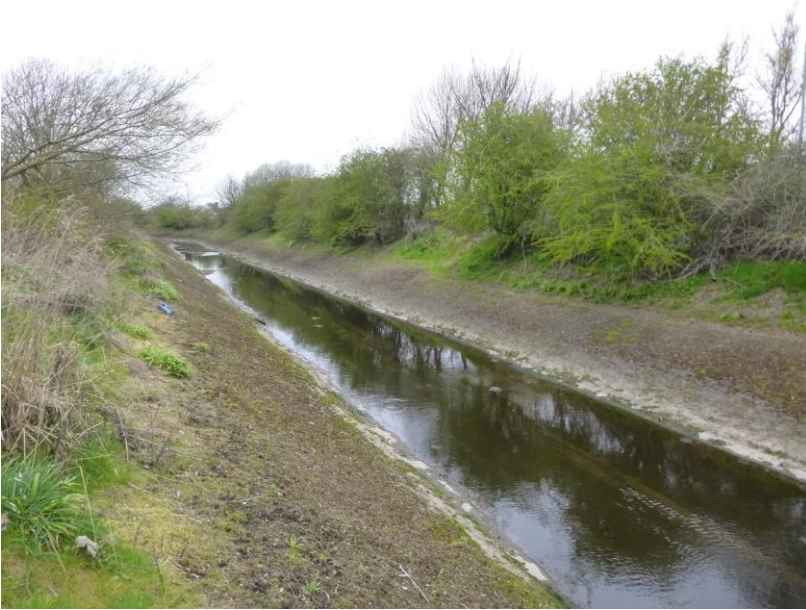
Photograph 2-6: Grange Burn flood relief channel adjacent to Wholeflats Road (NGR NS 93584 79999).
