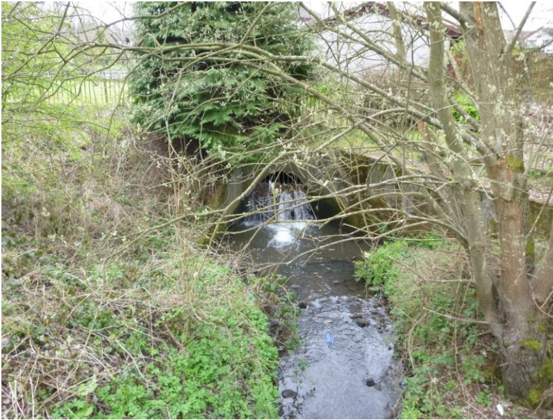
Photograph 2-3: Mungal Burn culvert (NGR NS 88205 82330).
