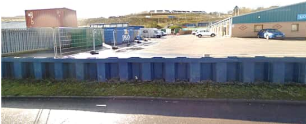
Figure 73: Sheet Pile example in Perth
