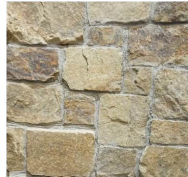
Figure 67: Sandstone type wall finish example
