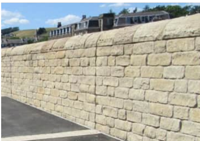
Figure 68: Stone wall with copes (Hawick)
