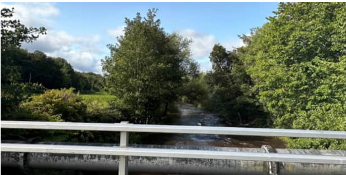
Figure 11: Photo 2 - View looking West along the River Avon at Jinkaboot bridge
