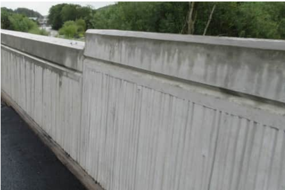
Figure 70: Example of a formed concrete wall
