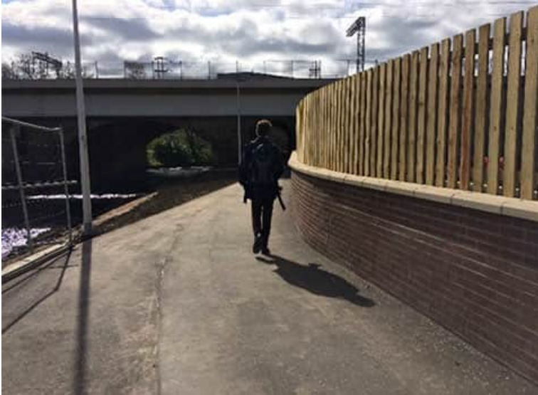
Figure 69: Brick flood wall in Edinburgh
