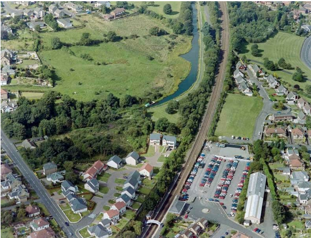
Figure 39: Photo 1 - Aerial view north-west of Falkirk High Station and the Union Canal (P57406, Falkirk Archives)
