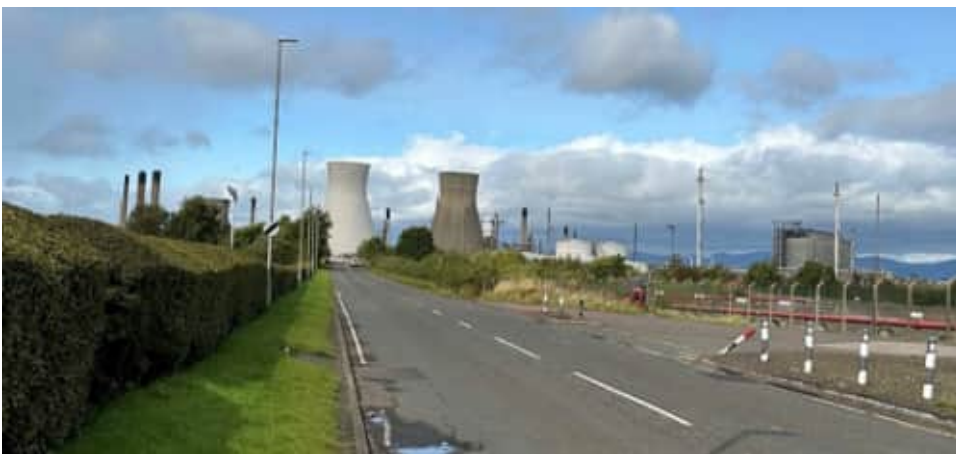
Figure 62: Photo 2 - View from A904 looking north
