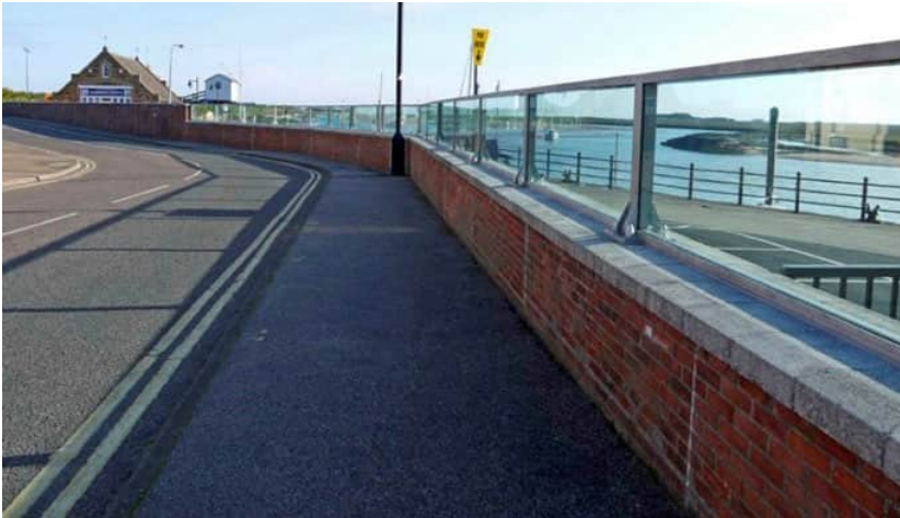
Figure 74: Example of glass flood barriers in Wells-next-the-sea (© Flood Control International ltd)
