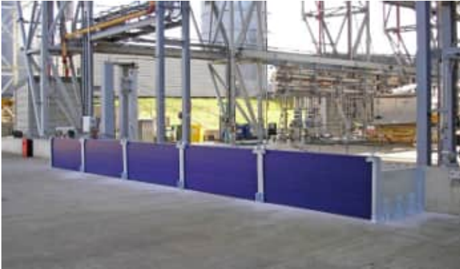
Figure 81: Removable Gate (© Flood Control International ltd)
