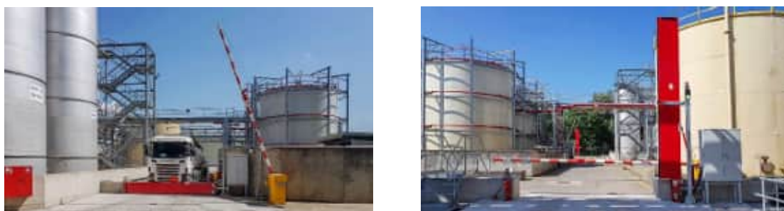
Figure 79: Pivot Flood Gate (© Flood Control International ltd)
