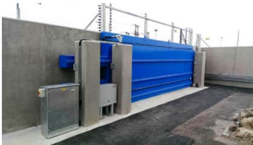
Figure 80: Heavy Duty Sliding Gate (© Flood Control International ltd)
