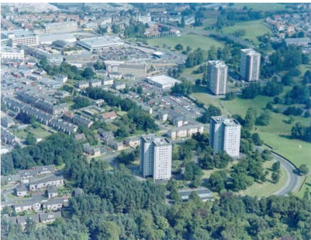
Figure 40: Photo 2 - Aerial view looking west over East Bridge Street and Callendar Park (P57473, Falkirk Archives)
