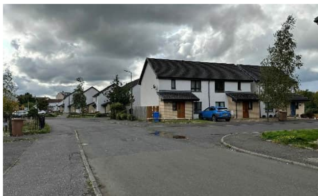
Figure 35: Photo 2 –Typical new housing estate
