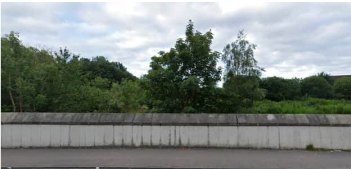
Figure 12: Plain concrete wall example
