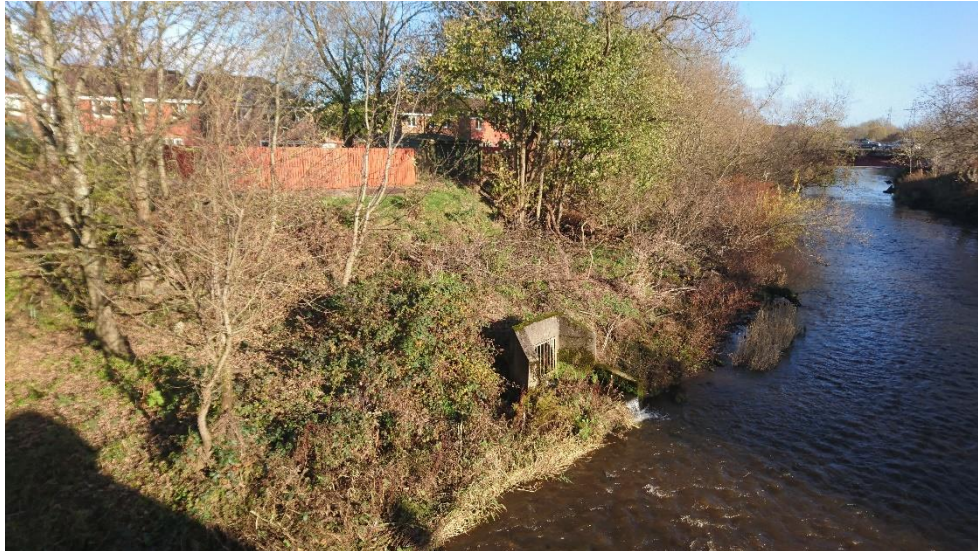
Figure 9-42: Photo 1-10 – View east from Stenhouse Road bridge
