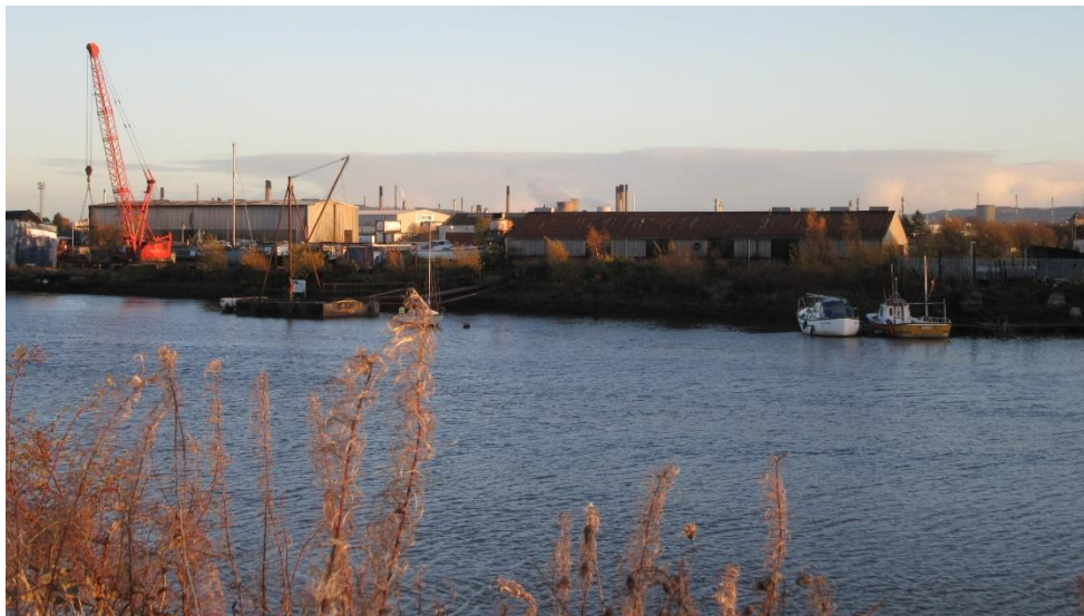
Figure 9–55: Photo 2-2 – View south from Core Path 006/024 to the Flood Cell area
