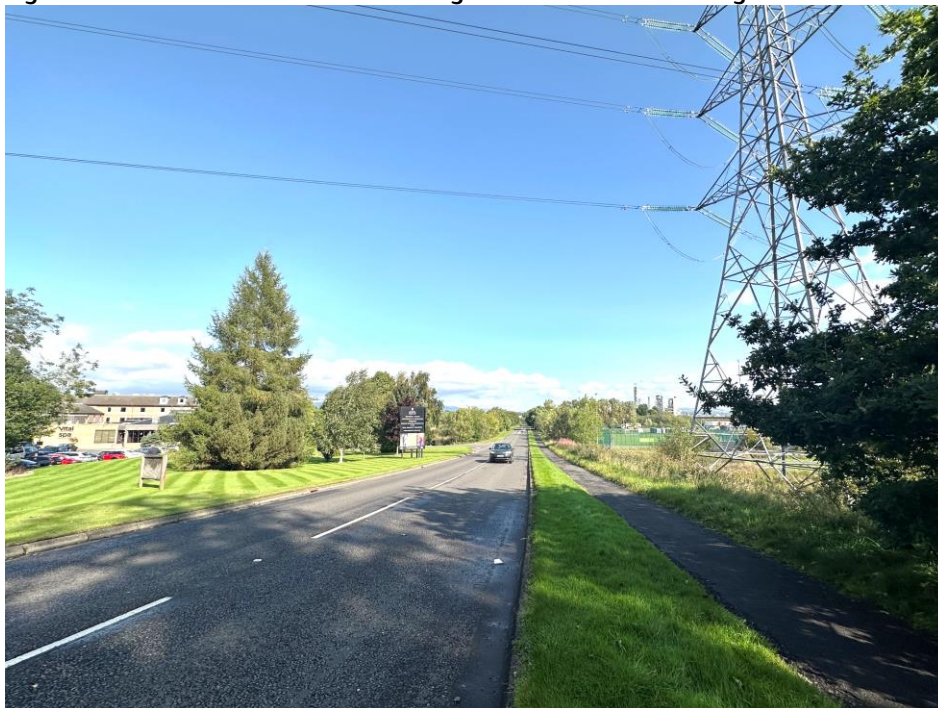
Figure 9-76: Photo 4-11 – View looking north on Grange Road (adjacent to proposed Core Path 016/027) with MacDonald Inchyra Hotel and Galaxy Sports playing pitches visible
