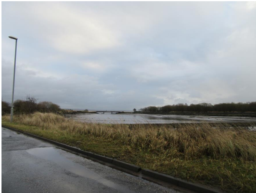
Figure 9–60: Photo 3-4 – View north-east along South Shore Road
