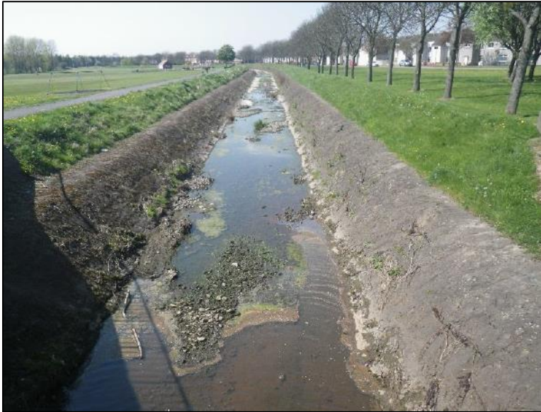
Figure 10-5: Grange Burn Flood Relief Channel (at Inchrya Park).
