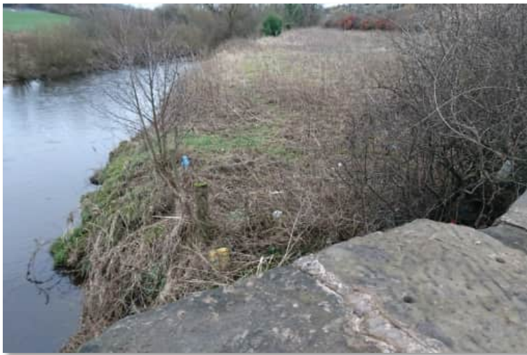
Figure 3-46: View looking east at bridge C51/20 (GR: NS 94781 79722)
