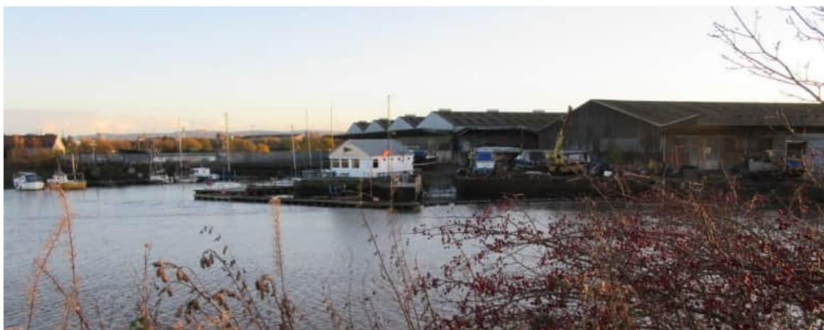
Figure 3-15: View looking east toward industrial buildings and Grangemouth Marina (GR: NS 92272 82651)
