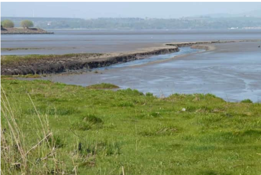
Figure 3-54: View looking northwest over the cooling water outfall channel (GR: NS 95312 82197)
