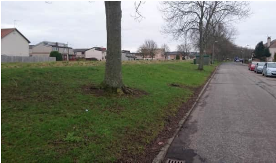
Figure 3-42: View south along existing embankment at Burnbank Road (GR: NS 92654 80547)
