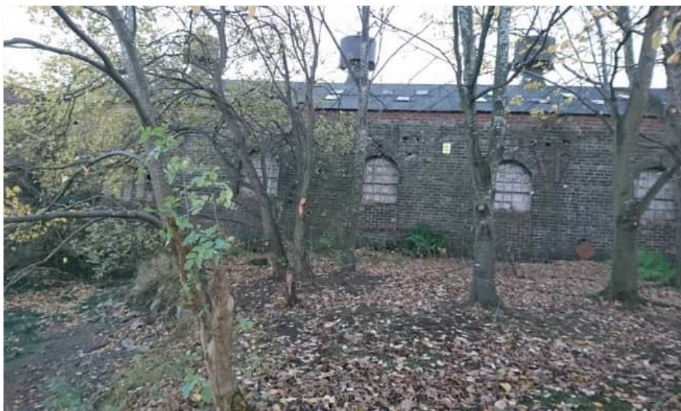
Figure 3-14: View looking east toward building that may be demolished (GR: NS 91807 82244)
