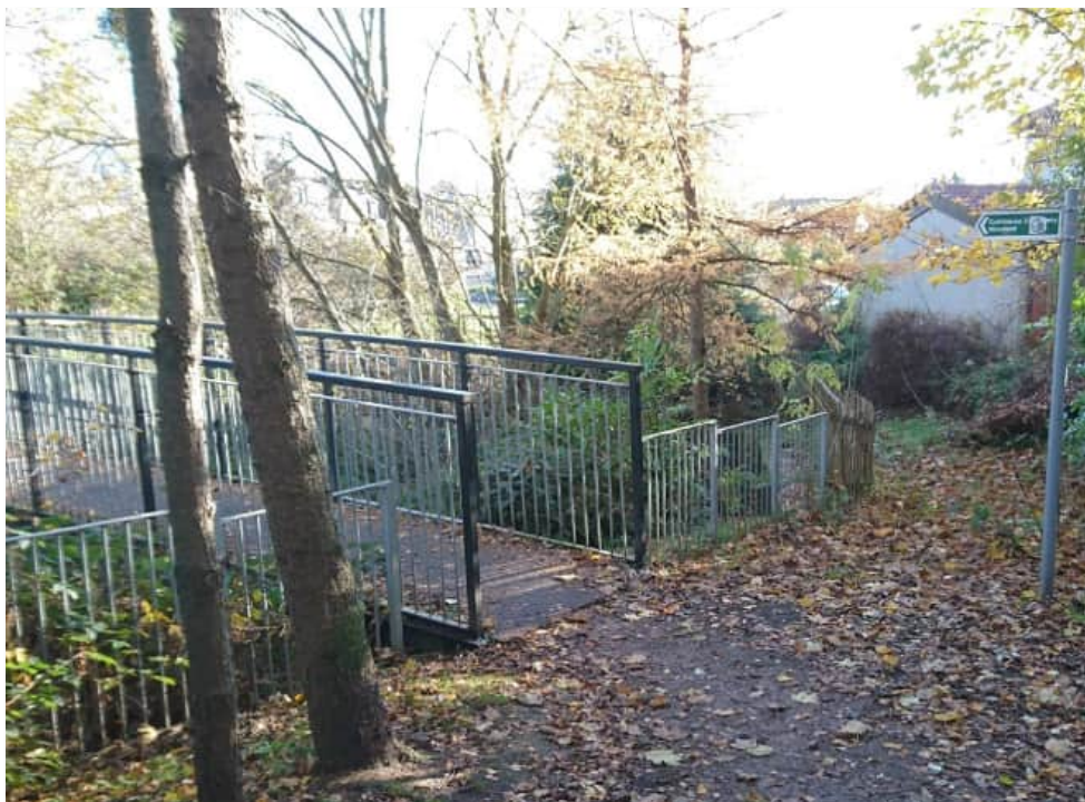
Figure 3-7: View looking southeast toward outlet of culverted watercourse (GR: NS 88193 82328)
