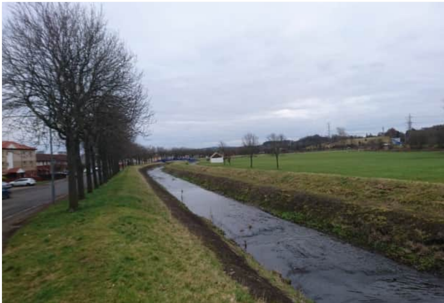
Figure 3-43: View looking east along existing embankment at Rannoch Park (GR: NS 92730 79892)
