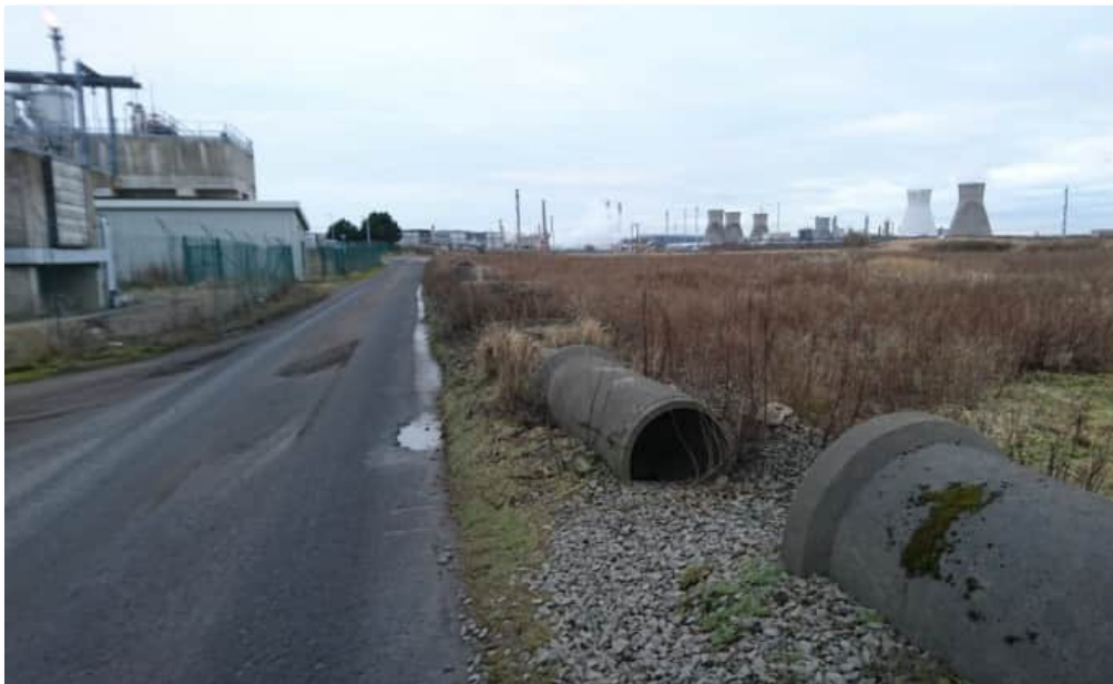
Figure 3-58: View looking south along defence alignment at sewage plant (GR: NS 96139 81188)
