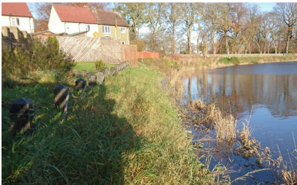
Figure 3-11: View looking northeast along rear of properties at Carron (GR: NS 89491 82920)
