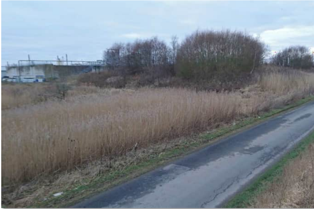
Figure 3-57: View looking southwest toward existing embankment and sewage plant (GR: NS 96313 81086)
