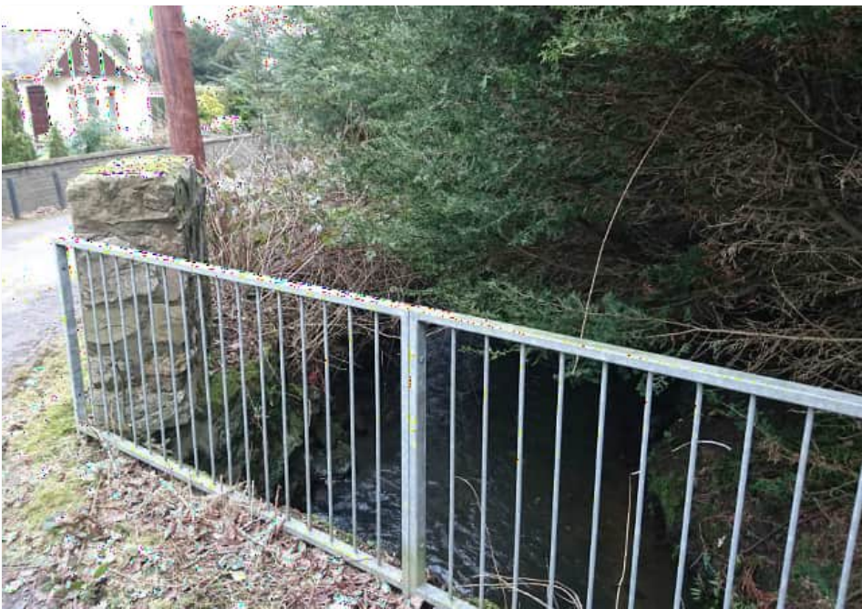
Figure 3-29: View looking east along Millhall Burn at Reddoch Road (GR: NS 94286 79619)
